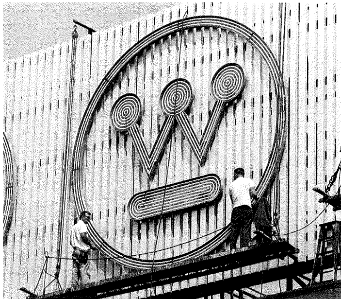
Fig. 34a: Installation of specialty signing.
